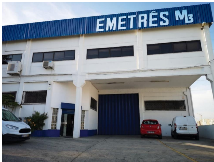
EMETRES Facilities in Lisbon, Portugal
