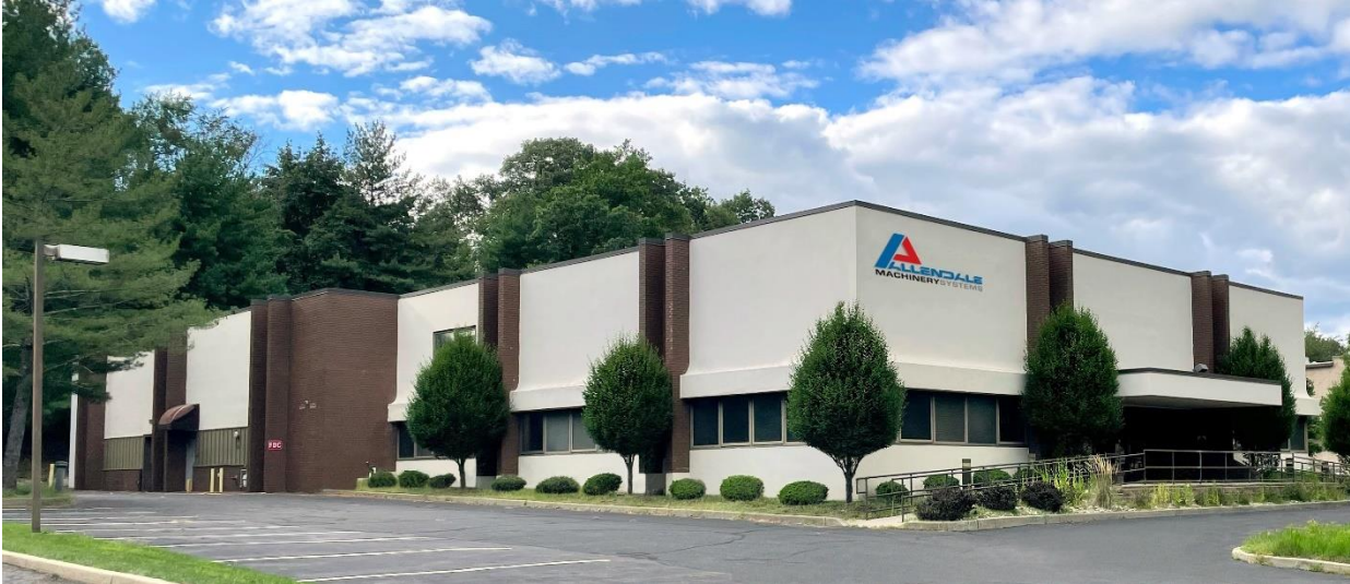
Allendale Machinery Systems Facilities in New Jersey
