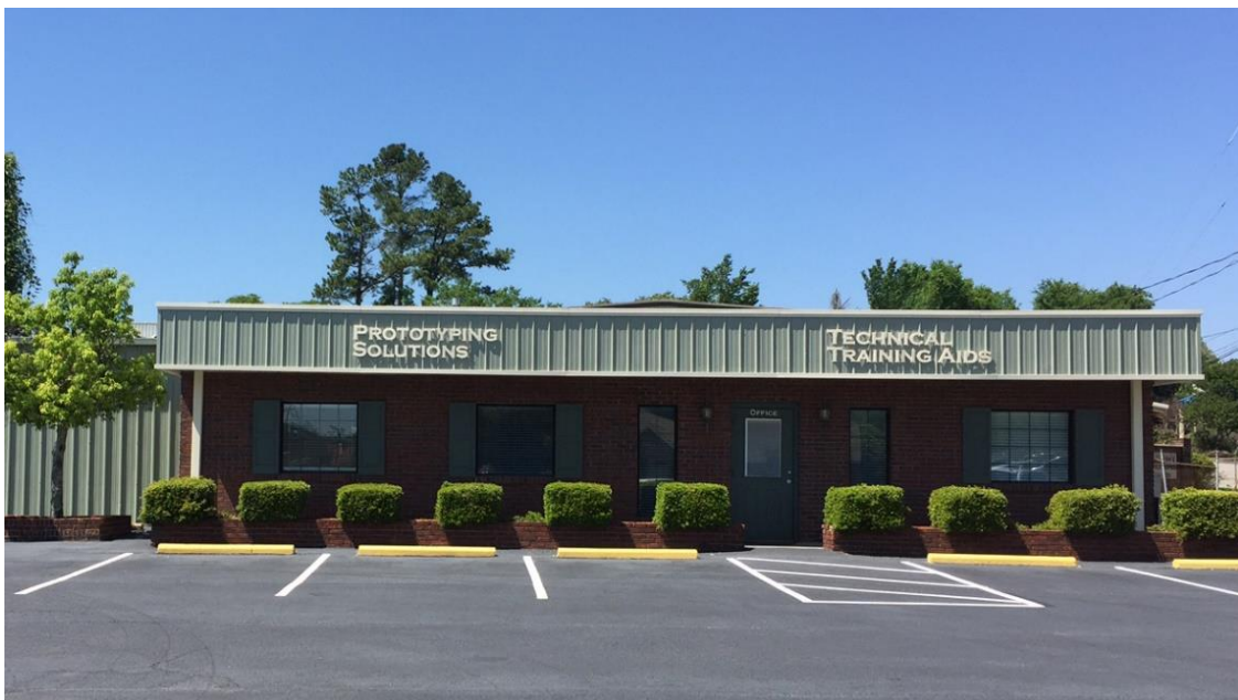
TTA and PS Facilities in Birmingham, Alabama
